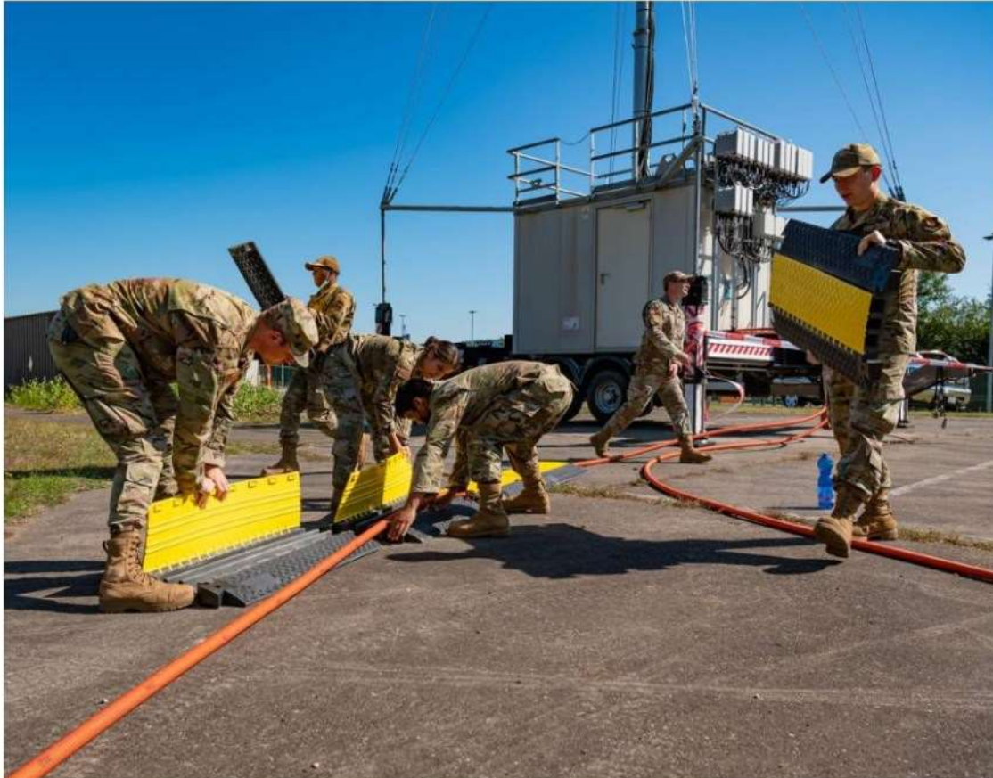
U.S. Air Force Airmen place protection around the inner ducts for the fiberoptic cables connected to a 5G cell tower at Ramstein Air Base, Germany, in 2021. NATO officials are monitoring 5G developments to harness new military benefits. (U.S. Air Force photo by Airman Jared Lovett)
