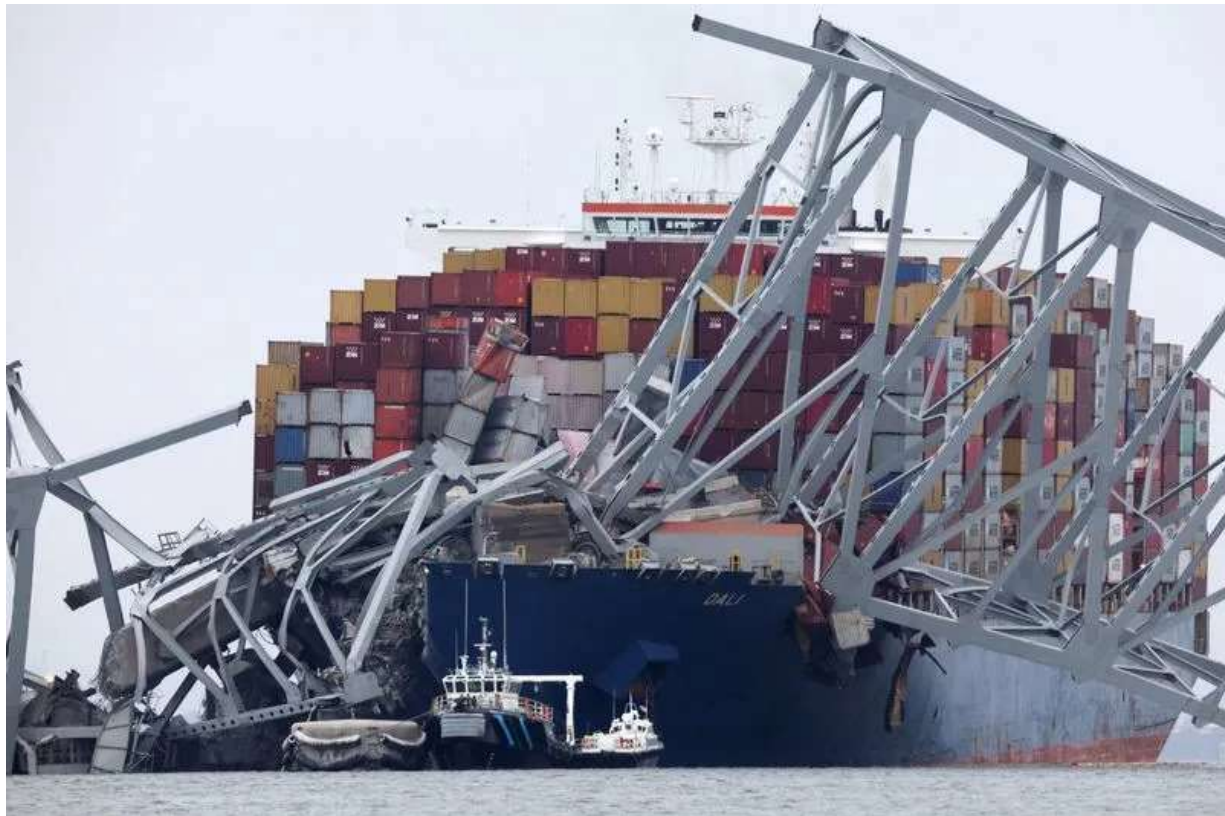
Francis Scott Key Bridge collapse in Baltimore
